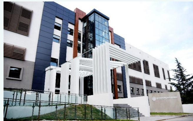
After Renovation October 2017
