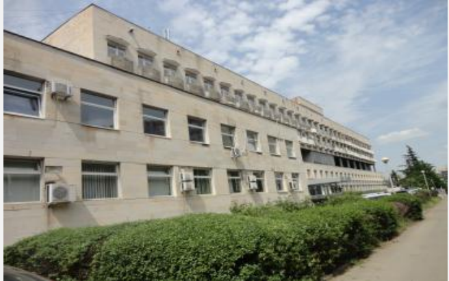
Before Renovation January 2016
