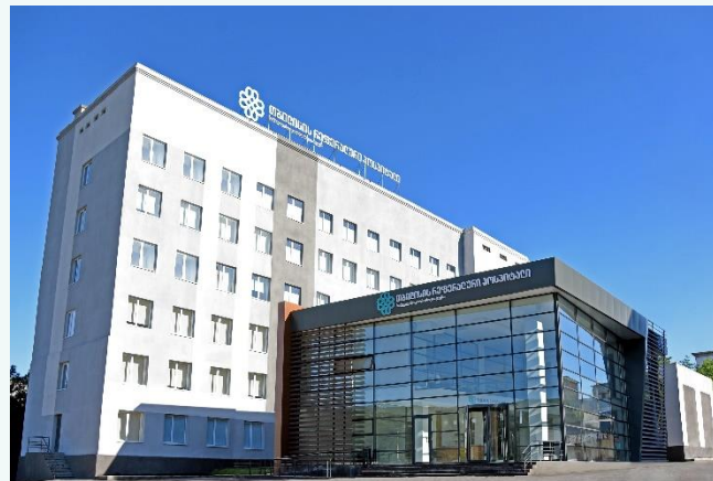
After Renovation October 2017
