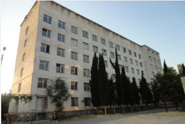
Before Renovation January 2016
